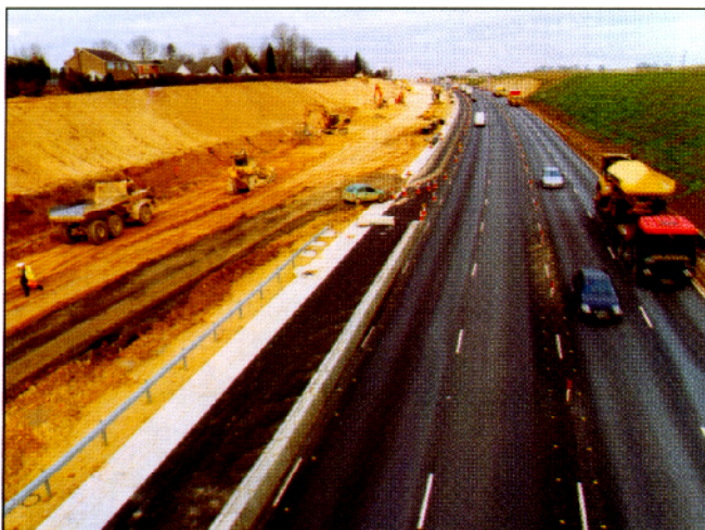
Above: A1 Northbound Carriageway Under Construction
