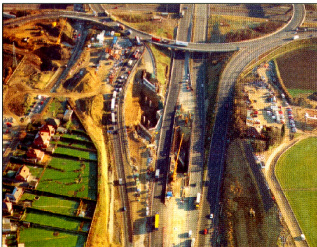
Above: M62 Tunnel Construction, Lothouse
