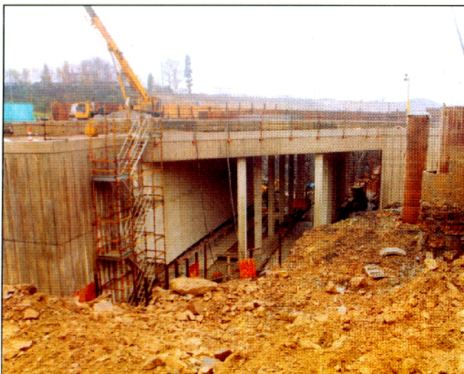
Above: M62 Tunnel, Lofthouse
