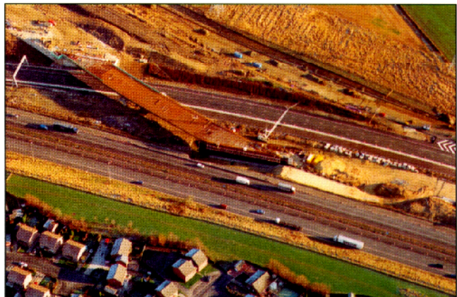
Above: St Georges Bridge, Belle Isle Interchange
